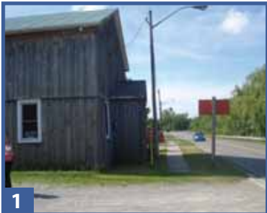
1 St. John's Parish Hall
