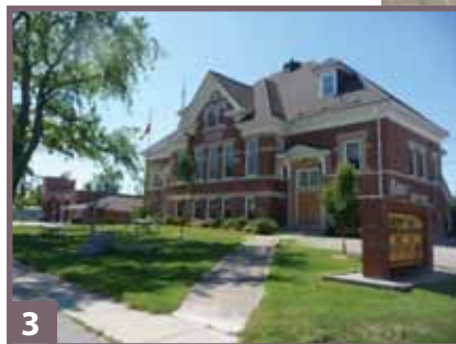
3 Selkirk Library and Community Centre
