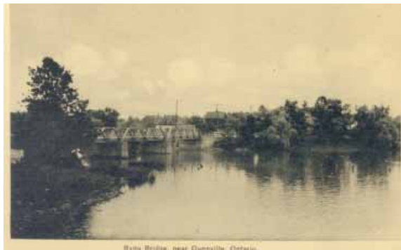
Byng Bridge (undated)
