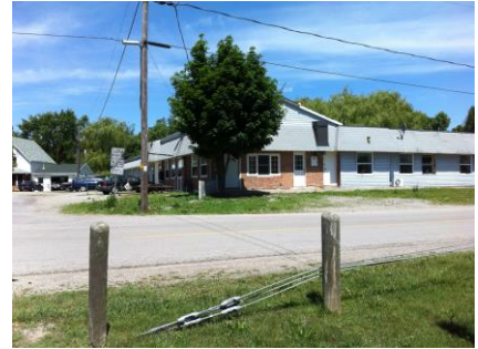
Commercial Roofed Accommodation in Port Maitland in need of exterior façade improvements
