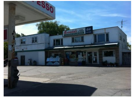
Byng gas station and garage in need of exterior improvements including signage. Redevelopment property
