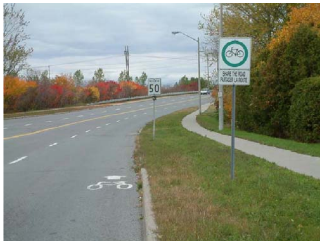
Wide Shared Use Lane, Ottawa, ON
