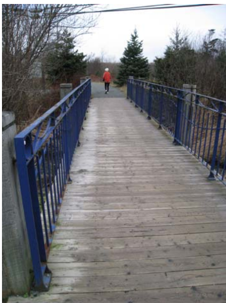
Trail bridge, St. John's, NFLD
