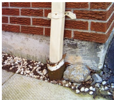
These downspouts are connected to the underground municipal sewer system.
