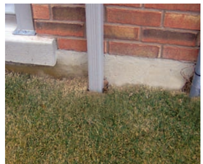
These downspouts are connected to the underground municipal sewer system.
