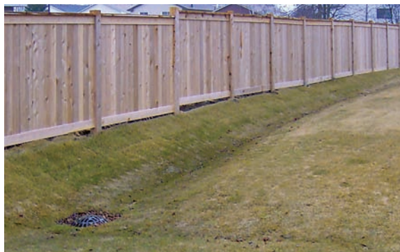
Rear-yard swales direct flows to a catch basin in this image. Rear-yard catch basins and swales shouldn't be covered or filled in with backyard sheds, fences or other structures, and rear-yard catch basins should be kept clear to reduce backyard flooding.
