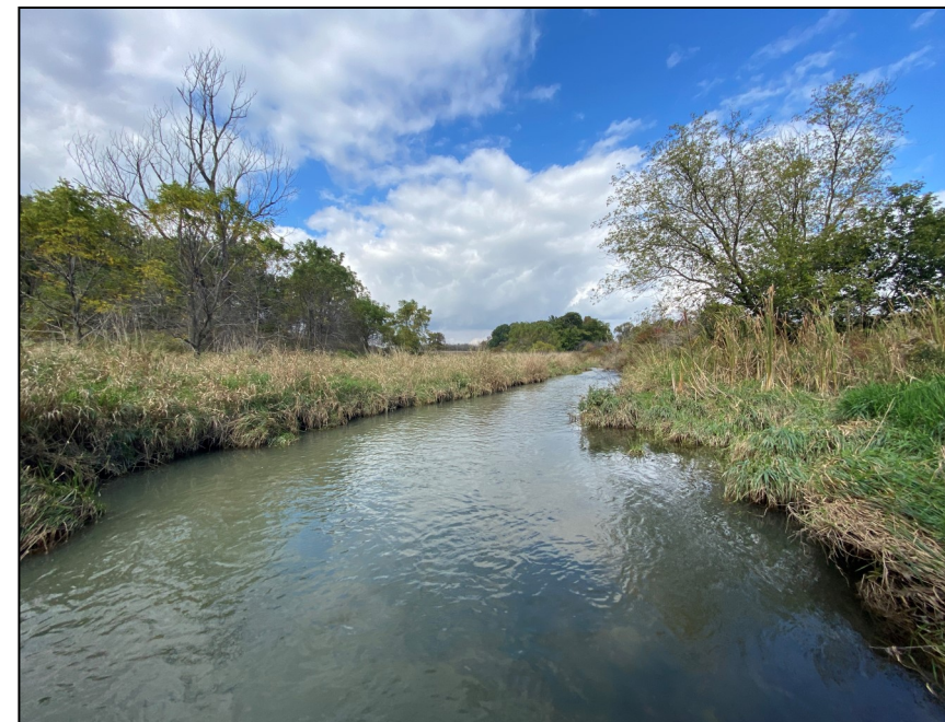
LEIP: Watercourse 2: Centre Creek at the box culvert of the New Lakeshore Road crossing – main channel. Looking upstream. October 13, 2021.
